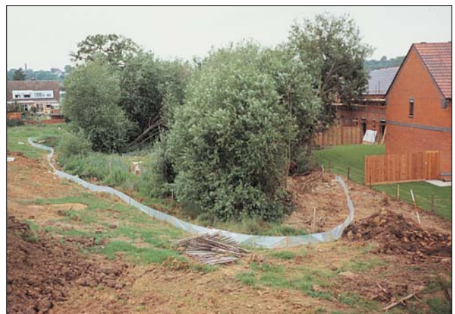
Drift fencing may be required to keep newts in agreed areas or to help in their capture and nearby release as a part of licenced mitigation schemes
